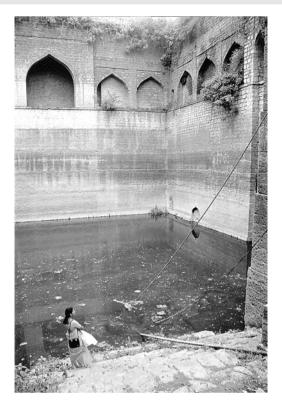
and 53 feet deep. There are octagonal domes on either side of the main gate with a parapet wall facing the entrance. The steps that commence from both the sides of the spacious halting rooms adjoin this wall and descend till the water level. There is a six-foot wide passage on three sides of the inner wall with resting places to the east, west and south built for the convenience of the travellers. One can have a full view of the *bavadi* from the gallery, which has arches engraved with motifs.
