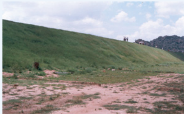
Rejuvenated tank bund
