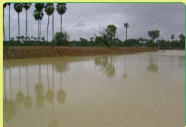
Pudhuvayal Kanmai after deepening
