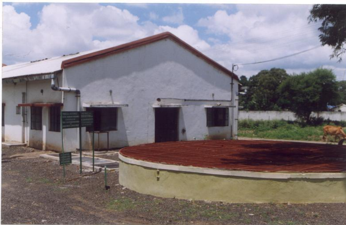
Fig 9 - Roof Top Rain Water Harvesting and Ground Water Recharge Through Dug Well at Musa Kheri, Indore Town, M.P.
