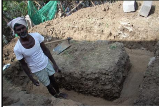
Foundation work is going on
