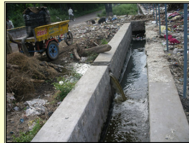
Discharging black water into open drain
