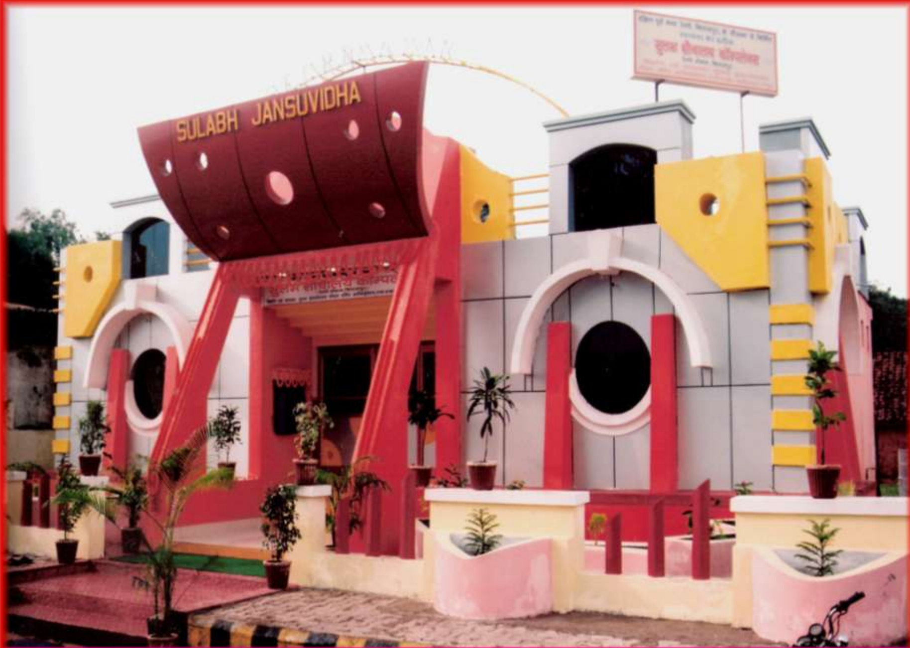
CONSTRUCTED SULABH TOILET COMPLEX AT CIRCULATING AREA OF BILASPUR RAILWAY STATION BY SOUTH EAST CENTRAL RAILWAY IN CHHATTISGARH
