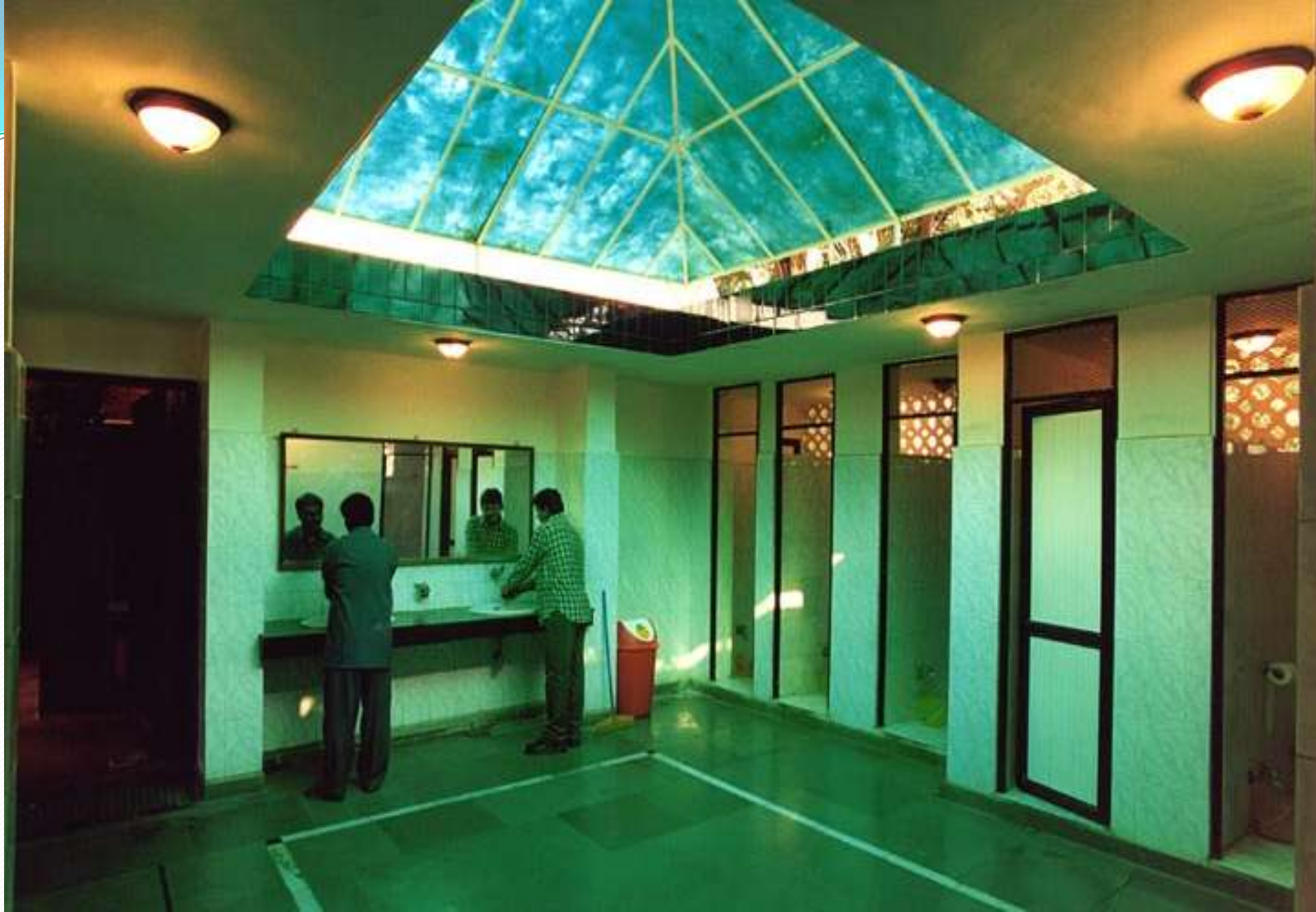
Wash Basin for Hand Wash – Inside view of Sulabh Toilet Complex, Delhi.
