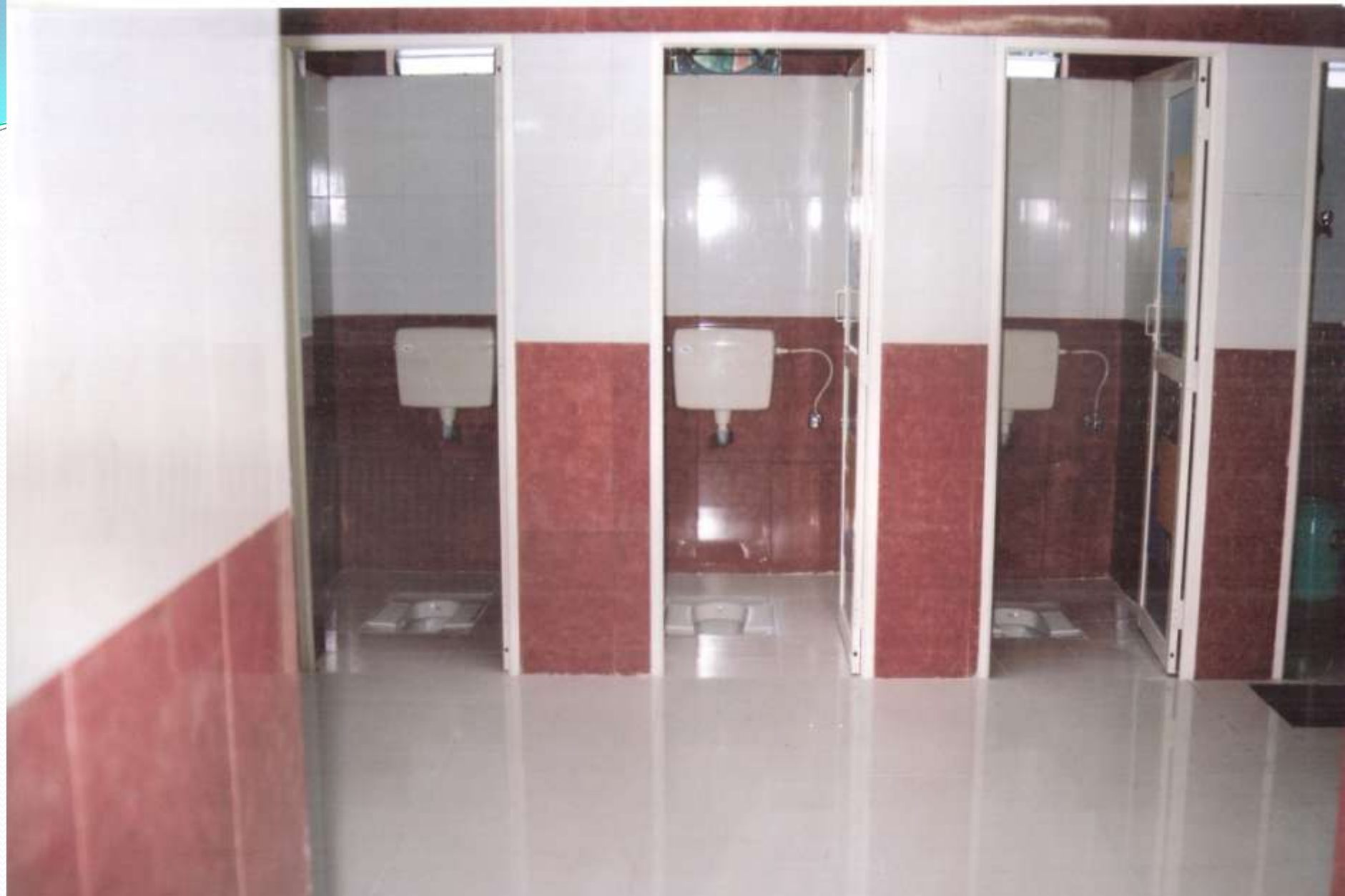
Inside View - Sulabh Toilet Complex, Bilaspur Railway Station, Chattisgarh
