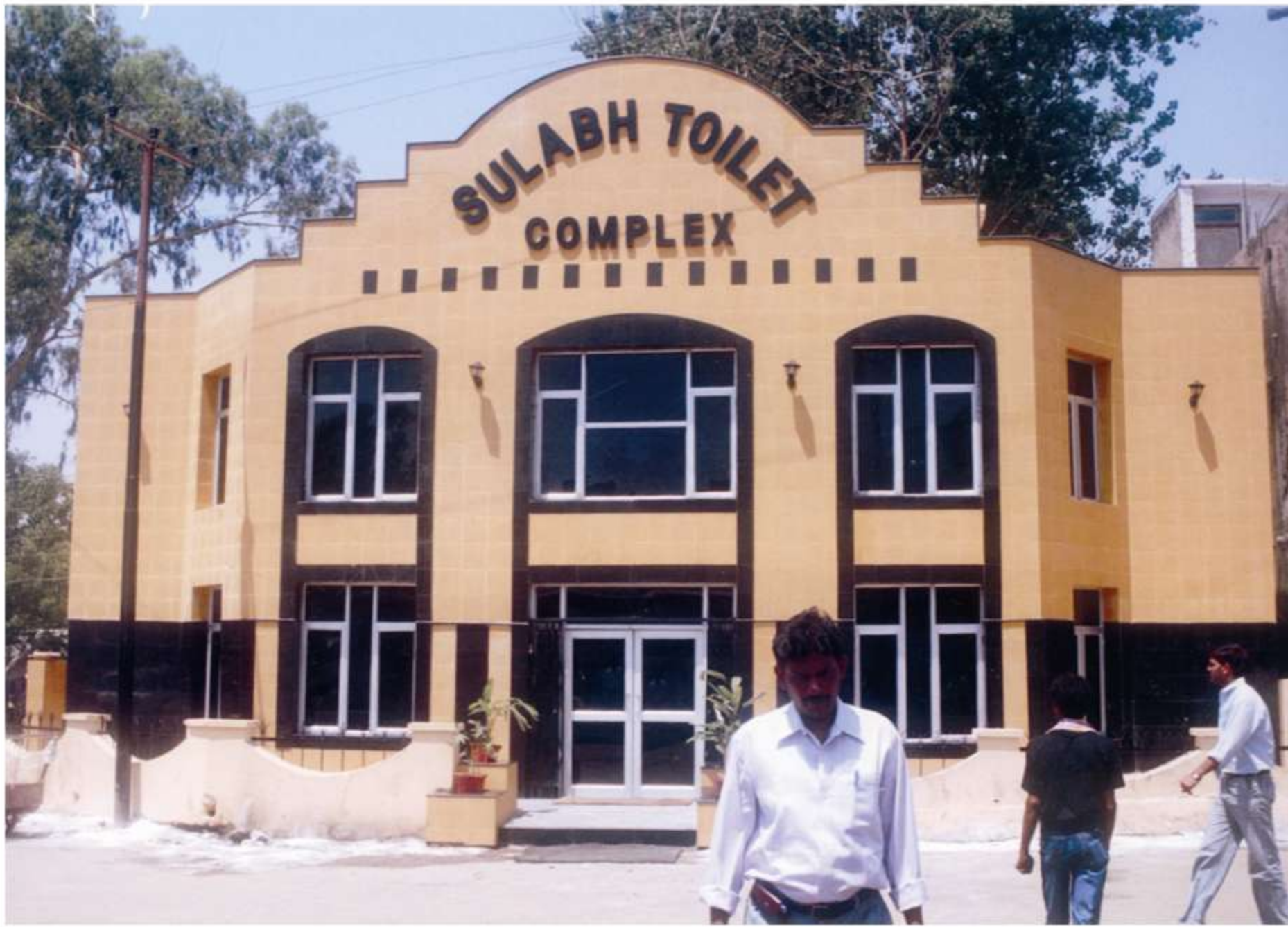
Sulabh Toilet Complex at Katra, Jammu & Kashmir.
