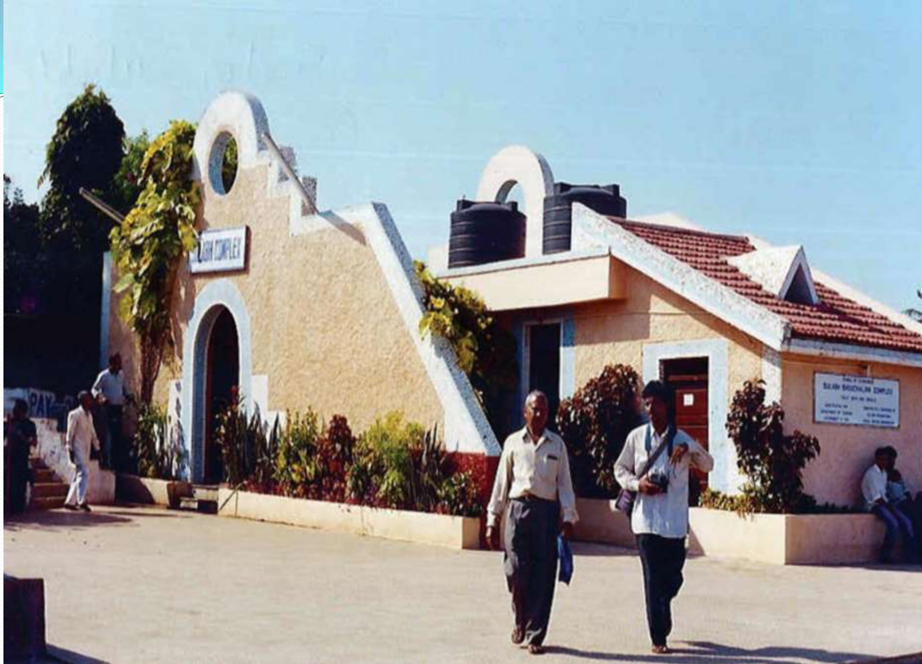
Sulabh Toilet Complex at Donapaula, Panji, Goa.
