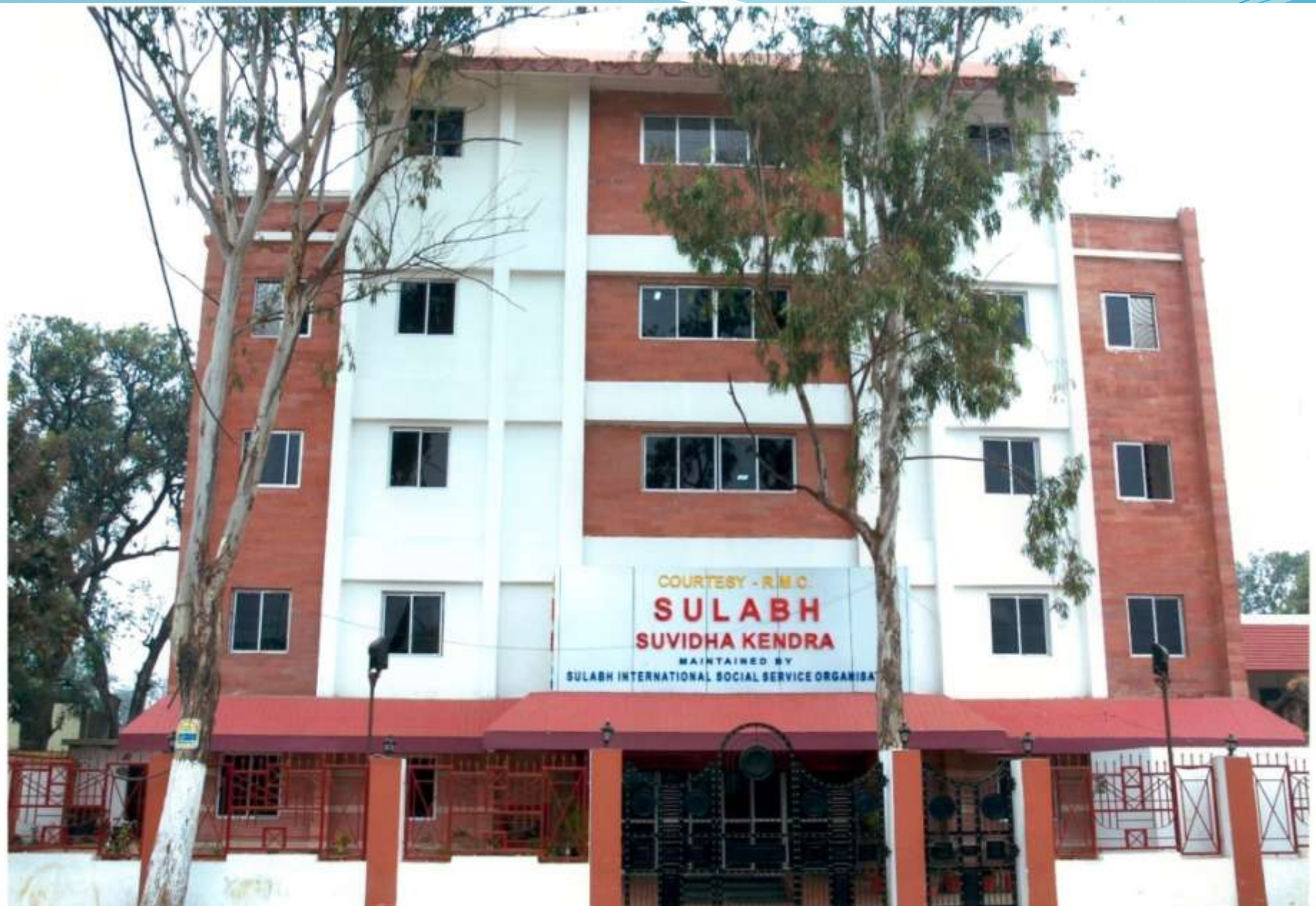
Sulabh Toilet Complex, Ratu Road, Ranchi, Jharkhand
