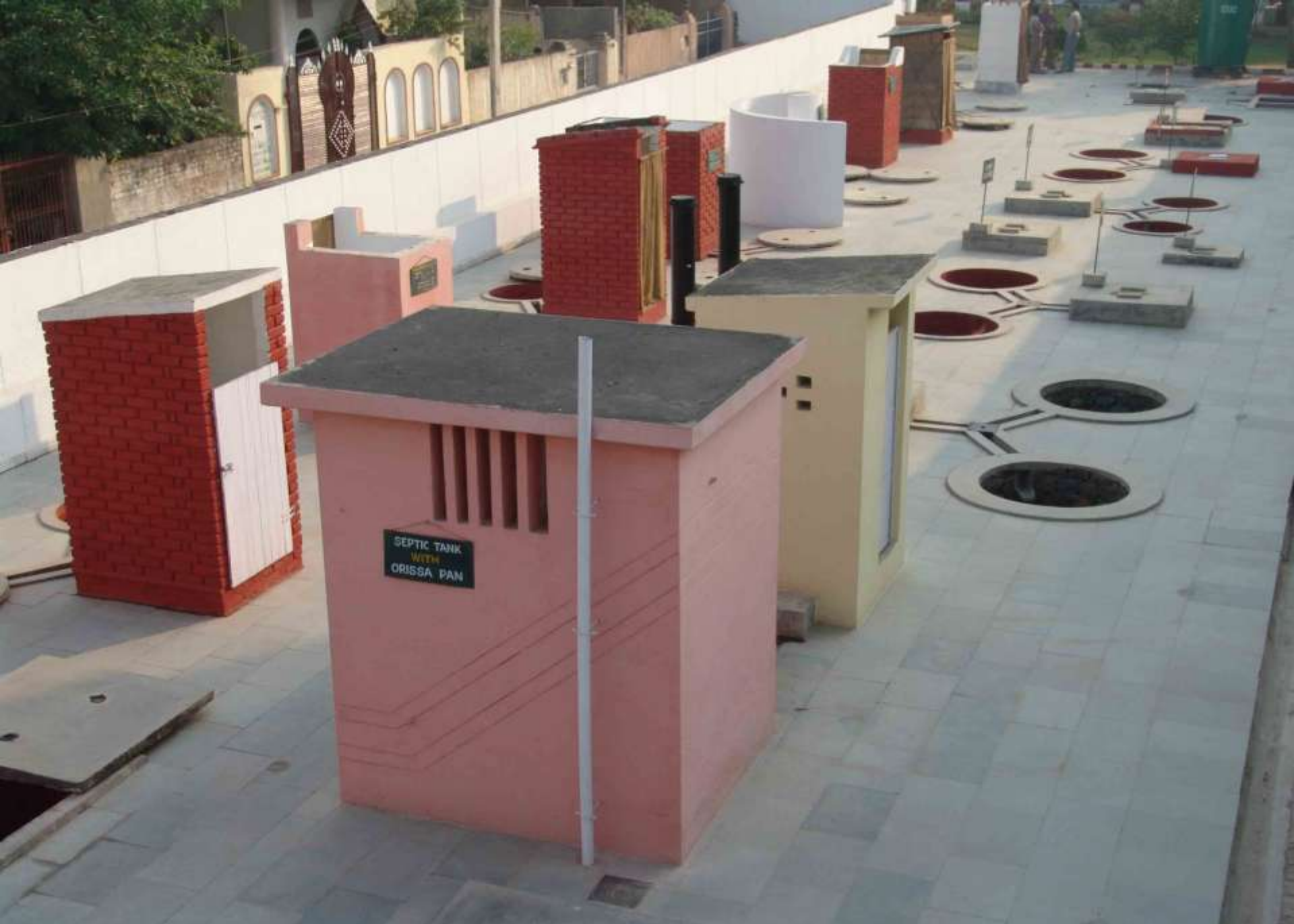
Panoramic View – Different Designs of Sulabh Two-Pit Pour Flush Compost Toilets
