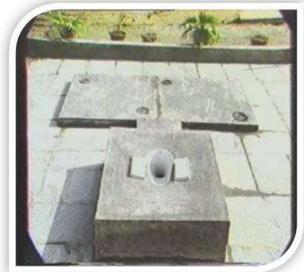
Sulabh Toilet with rectangular pits.
