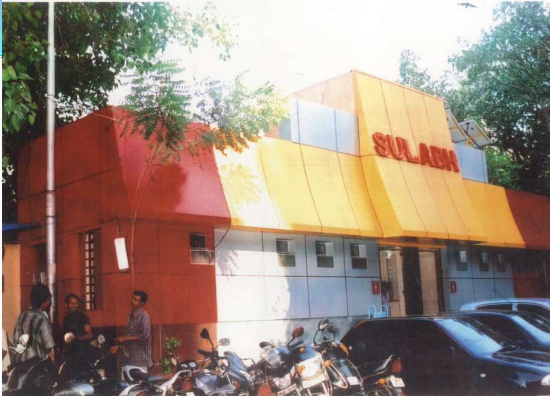
Sulabh Toilet Complex - Premium Business Centre, Nariman Point,, Mumbai
