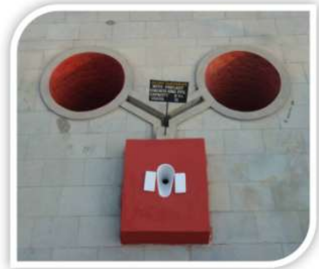
Sulabh Toilet with circular pits.
