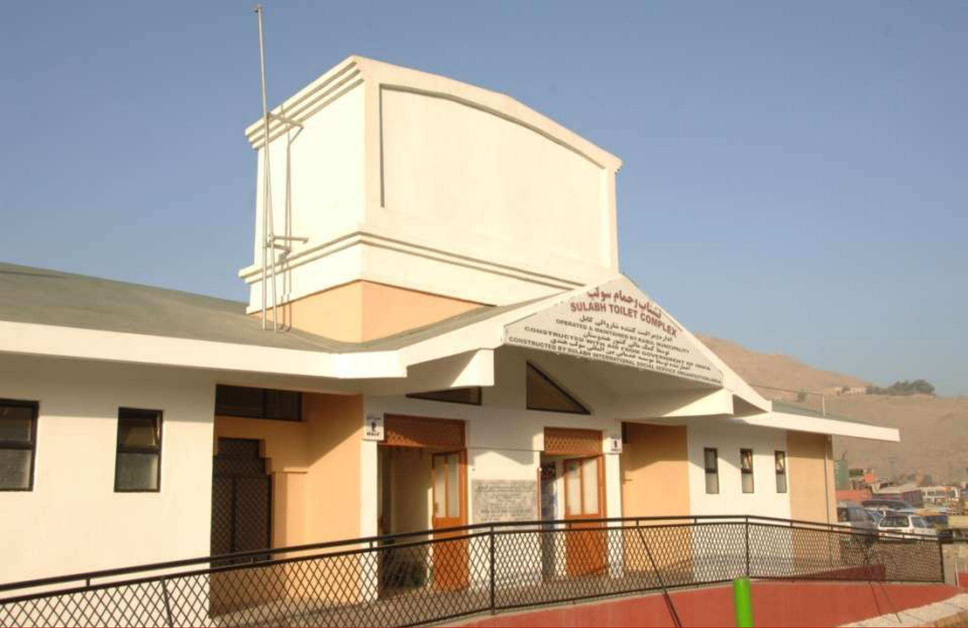
Sulabh Toilet Complex at Kabul, Afghanistan
