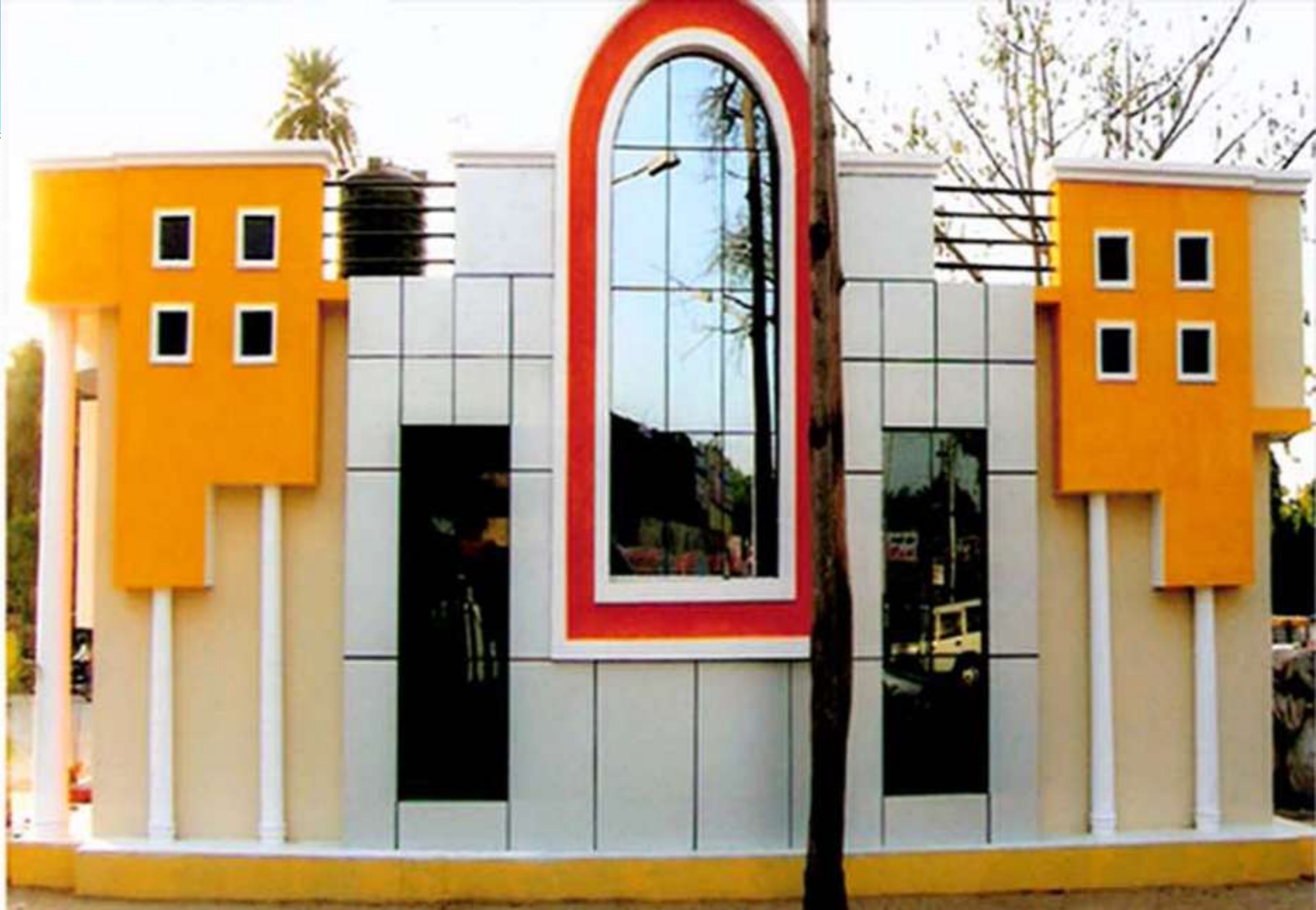
Sulabh Toilet Complex, Rewa, Madhya Pradesh
