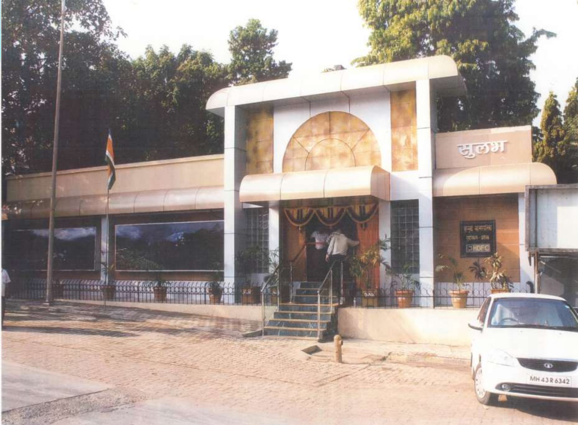
Sulabh Toilet Complex – Andheri Kurla Metro Rail, Mumbai
