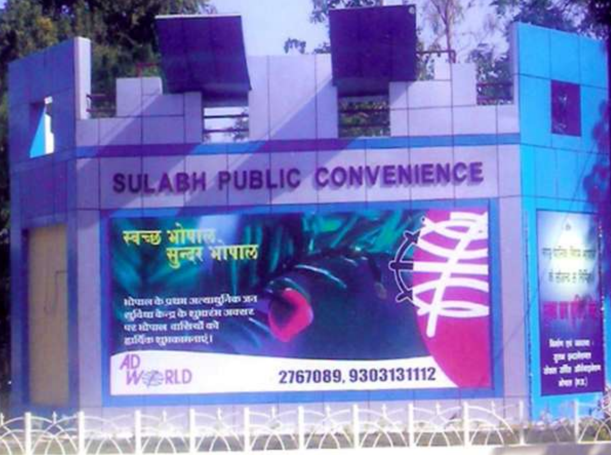
VIEW OF HI-TECH SULABH TOILET COMPLEX AT 10 NO BUS STOP , BHOPAL DURING 2005-06
