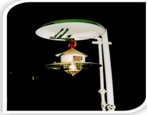
Biogas used for lighting of mantle lamps
